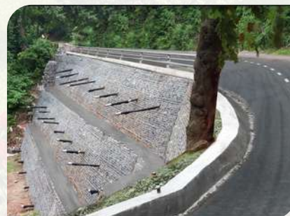
Soil Nailed Slope Protection at Daringbadi
