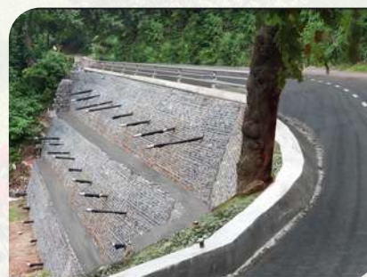
Soil Nailed Slope Protection at Daringbadi
