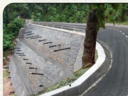
Soil Nailed Slope Protection at Daringbadi
