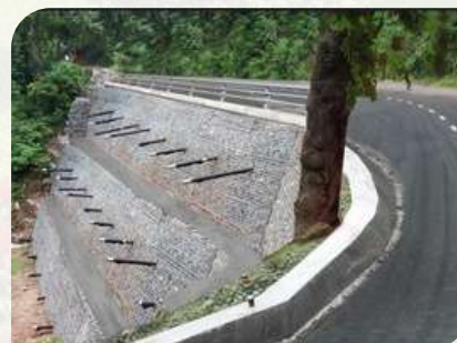
Soil Nailed Slope Protection at Daringbadi
